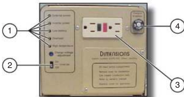
Figure 3-9. 800W AC Inverter Location
